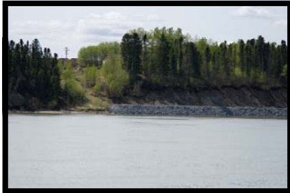
Shoreline Stabilization after picture
